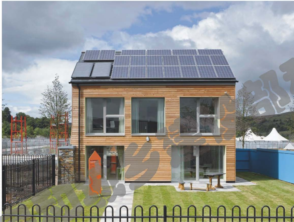
Examples of Solar Panels on a Passivhaus in Wales, UK.
